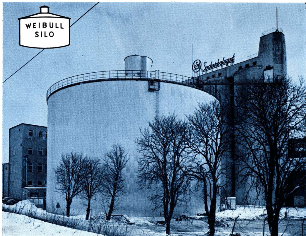
Above, a 10,000 ton white sugar silo built in 1933. It was enlarged in 1961 to take 30,000 tons.
