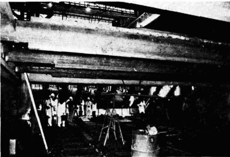
Inside the diffuser under construction at Amatikulu
