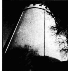
DDS Silo for storing white sugar in bulk.
