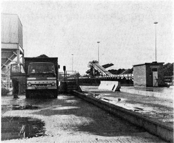
Fig. 1. A load of beet about to be tipped into receiving hopper. The beet then travels under the road via apron chain conveyors to the main belt system, and thence to the travelling boom stacker seen in the background.
