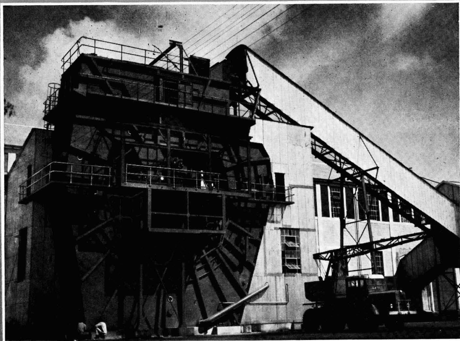
The Saturne diffuser at Saint-Antoine Sugar Factory (Mauritius)
