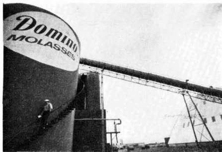
Molasses tank and pipeline at Amstar sugar refinery
