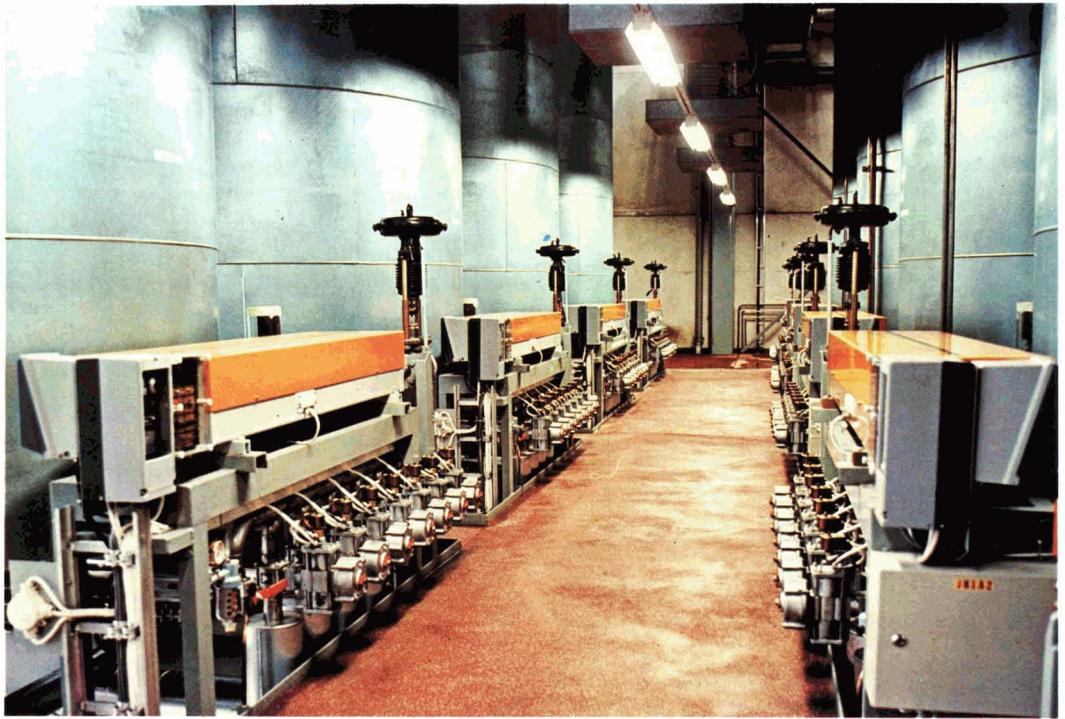
Molasses Desugarization Plant, Naantali Sugar Factory, Finland.
