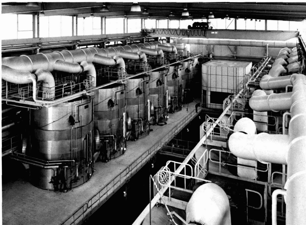
General view of a new boiling house for a capacity of 12,000 t/d. Technological, conception, layout and supervision of work carried out by IPRO.
