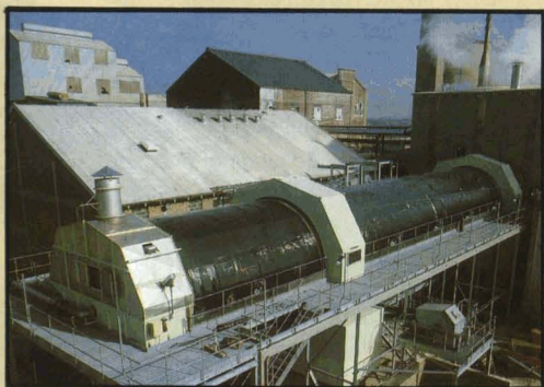
An RT5 Beet Diffuser capable of processing up to 4500 tonnes of beet per day recently installed and commissioned at BSC Brigg Factory England. (Photograph by permission of the British Sugar Corporation)
