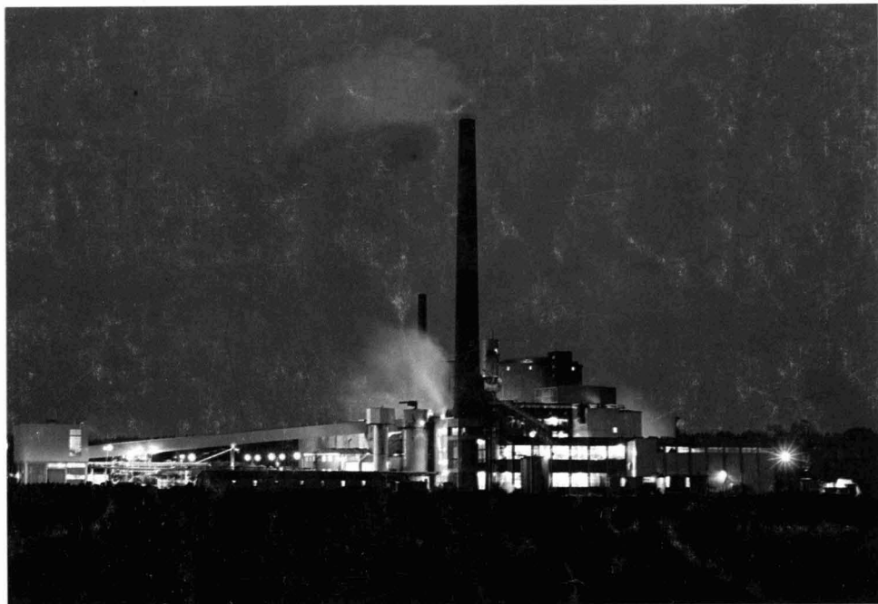
Braunschweiger Zucker AG, Wierthe Sugar Factory. Overall engineering design and supervision: IPRO
