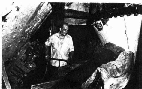
Fig. 14. Transfer of spent adsorbent from the old cisterns
