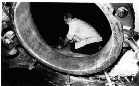
Fig. 12. Securing a blanket for the underdrain system of the old cistern
