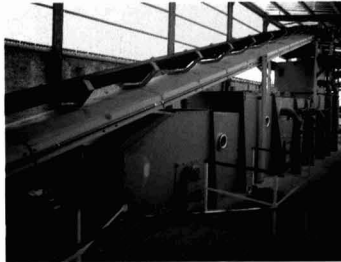
Savings of around 4 kg of fuel oil per tonne of beet processed.
