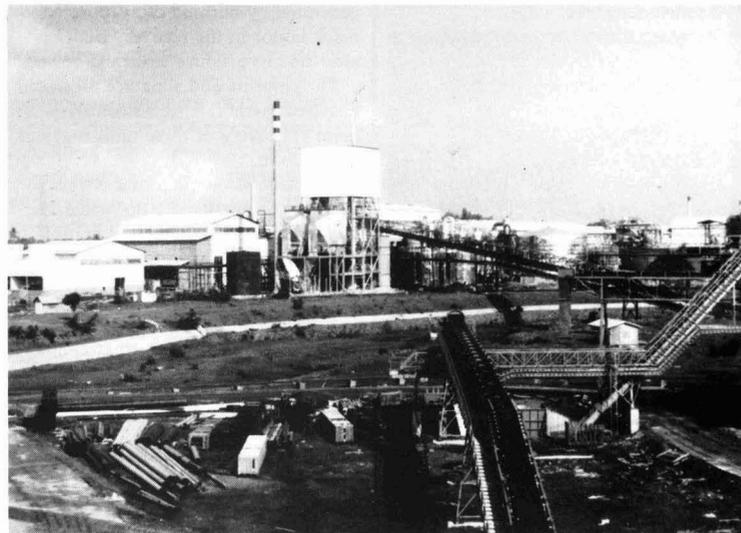
View of the recovery boiler, evaporation plant and pulp line
