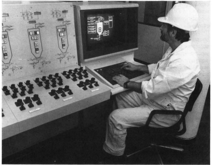
Figure 3. Process operator at a VDU in the wet process control room of Pyrmont Refinery
