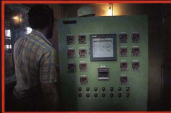
▲ Commissioning the control panel
