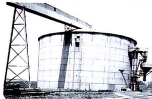
In 1933, Nils Weibull AB delivered the world's first steel silo for storage and handling of bulk products such as sugar.
