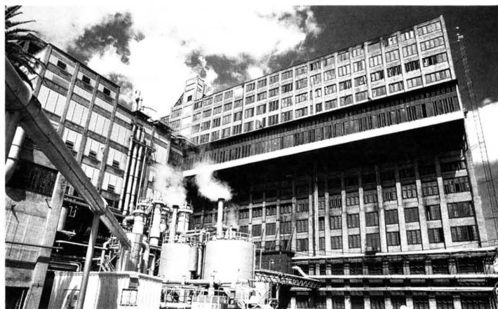
Carbonatation station (left-centre), filter/char house (background right) and pan house (background left)
