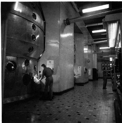
Figure 4. The pan floor at Thames refinery
