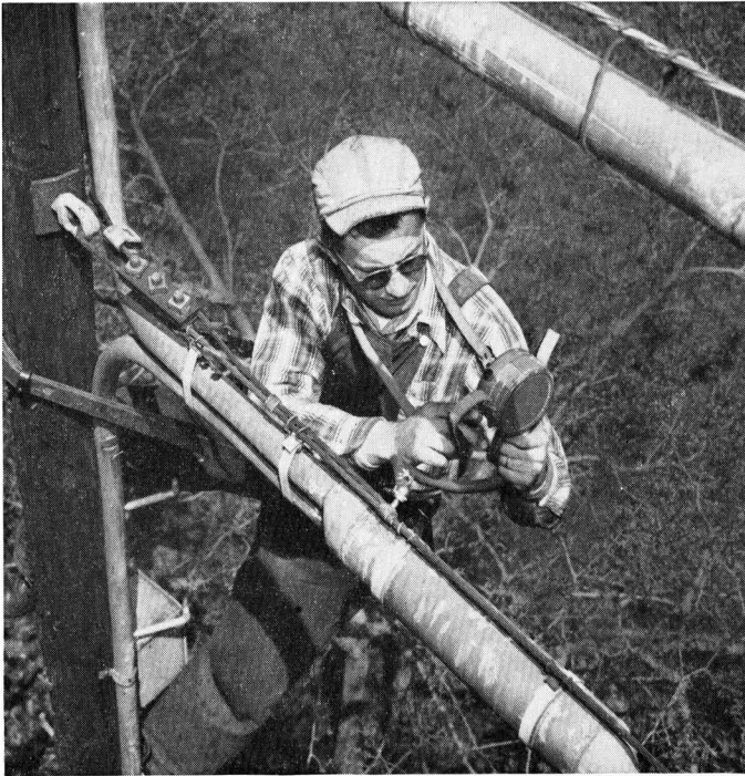
Air compressor and tank are at right. Long cylinders on rack dry air before it enters cables.
