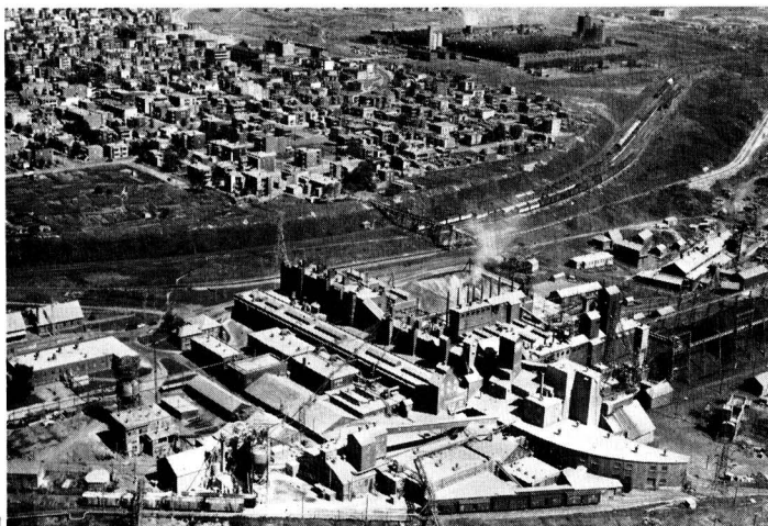
FIG. 4. The calcium carbide division of Shawinigan Chemicals Limited at Shawinigan Falls, Quebec, the largest producer of carbide in the British Commonwealth. It uses about 100,000 hp of electrical energy. Beside it, to the right, is the stainless steel and alloys division of the company.
