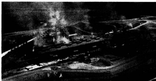
Aerial view of Monsanto Chemical Co.'s electric furnace elemental phosphorus plant at Monsanto, Tenn.
