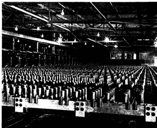
DeNora cell room, hub of Pennsalt's newest chlor-caustic plant at Calvert City, Ky.
