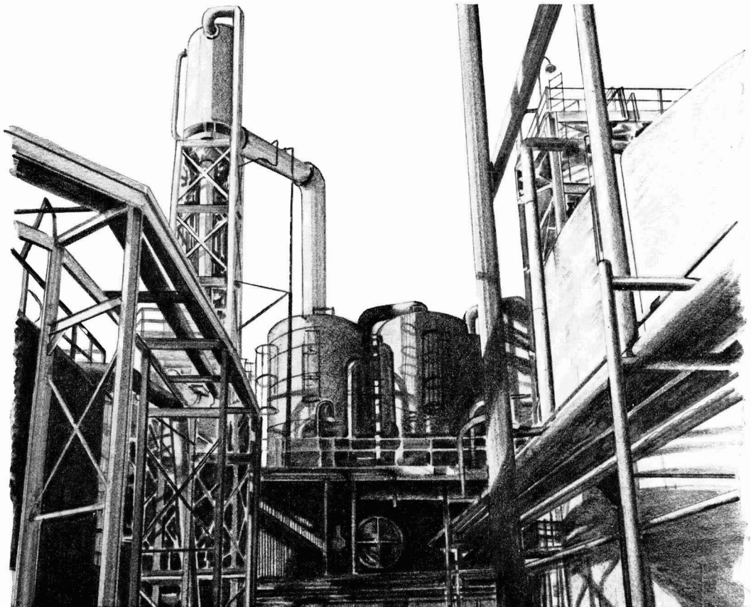
The Frontier Chlor-Alkali Plant at Wichita, Kansas
