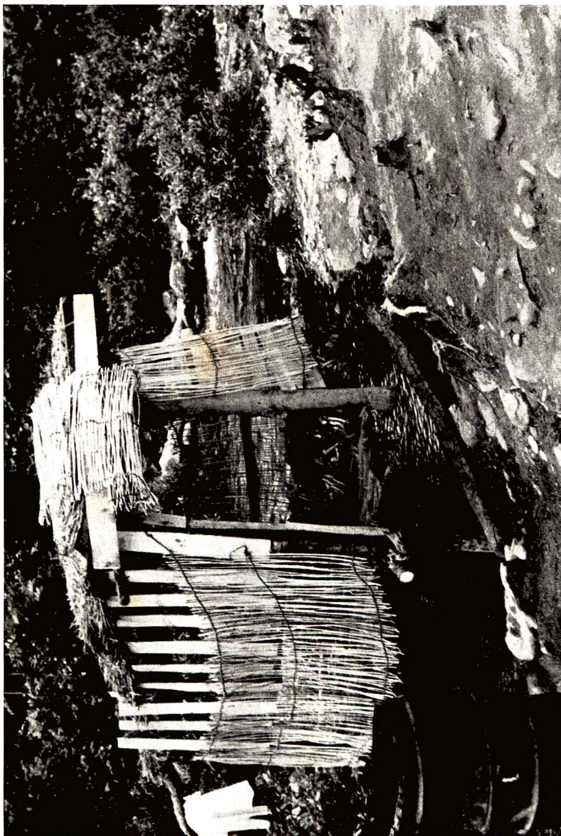
Fig. 6 A military mess storage cabinet for vegetables built over a creek to keep them cool.
