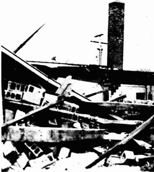
Roof collapse from snow accumulation
