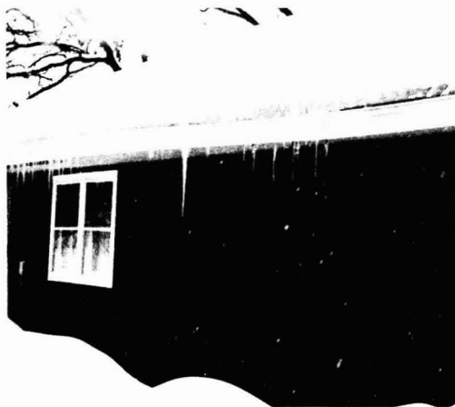
Conditions conducive to ice dam formation
