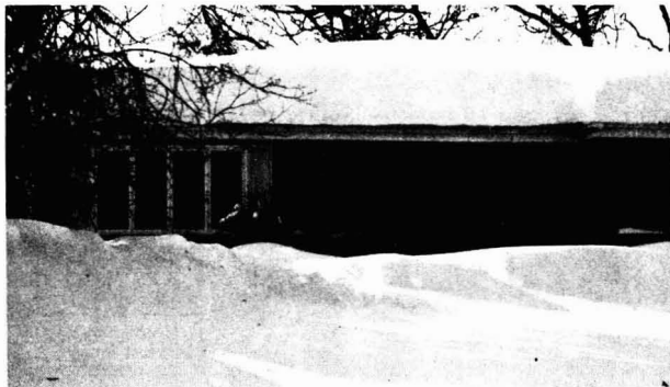
Snow accumulation on roof
