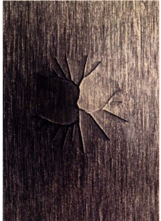
Coating without Hycar® RLP shows significant damage.
