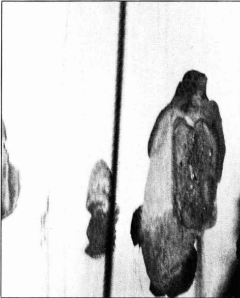
Figure 4 —The fourth stage of corrosion shows severe pitting and loss of steel. The lining has completely lost adhesion. Red rust is noted
