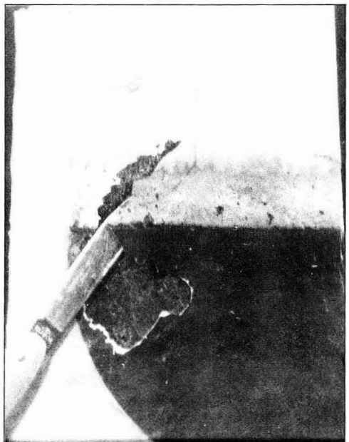
Figure 8—A 40 mil epoxy-amine system failed by delamination within 30 days
