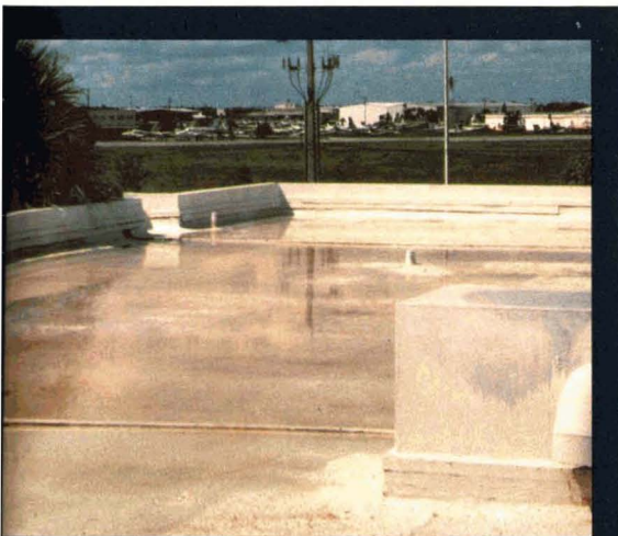
This roof in Florida demonstrates how a roof mastic based on RHOPLEX EC-1895 acrylic retains its initial integrity under ponded water conditions.
