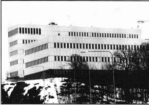
Figure 31—Plastisol coated steel panels. Office building, Uddevalla, Sweden, erected 1974
