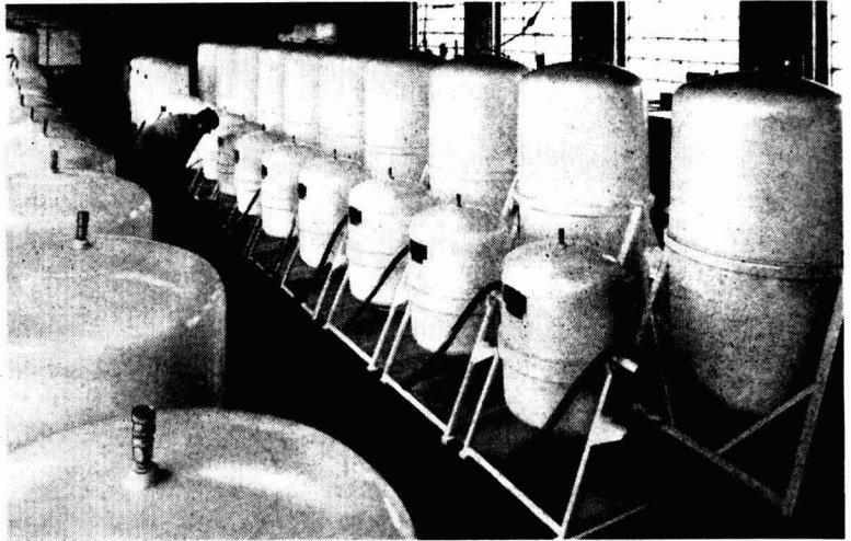
A recent installation of 36—360 gallon Portatanks at Joseph Mason & Co. Limited Derby
