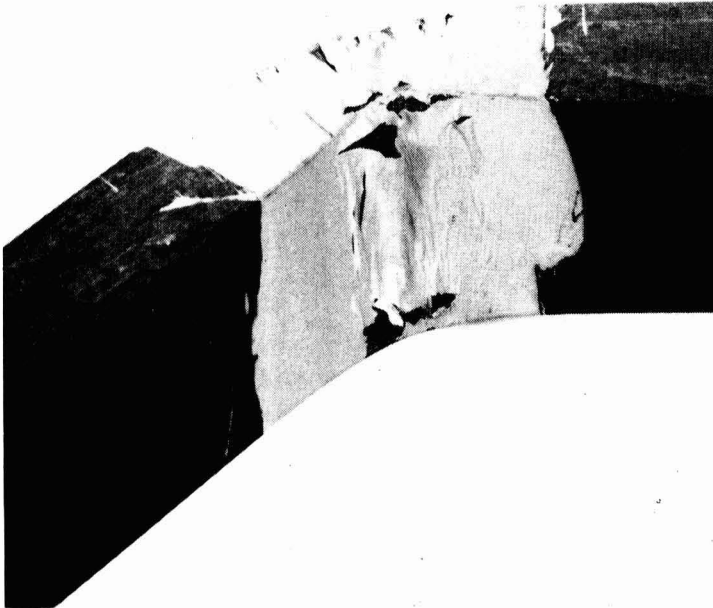
Fig. 4. Paint failure on a bent beam; compressive face
