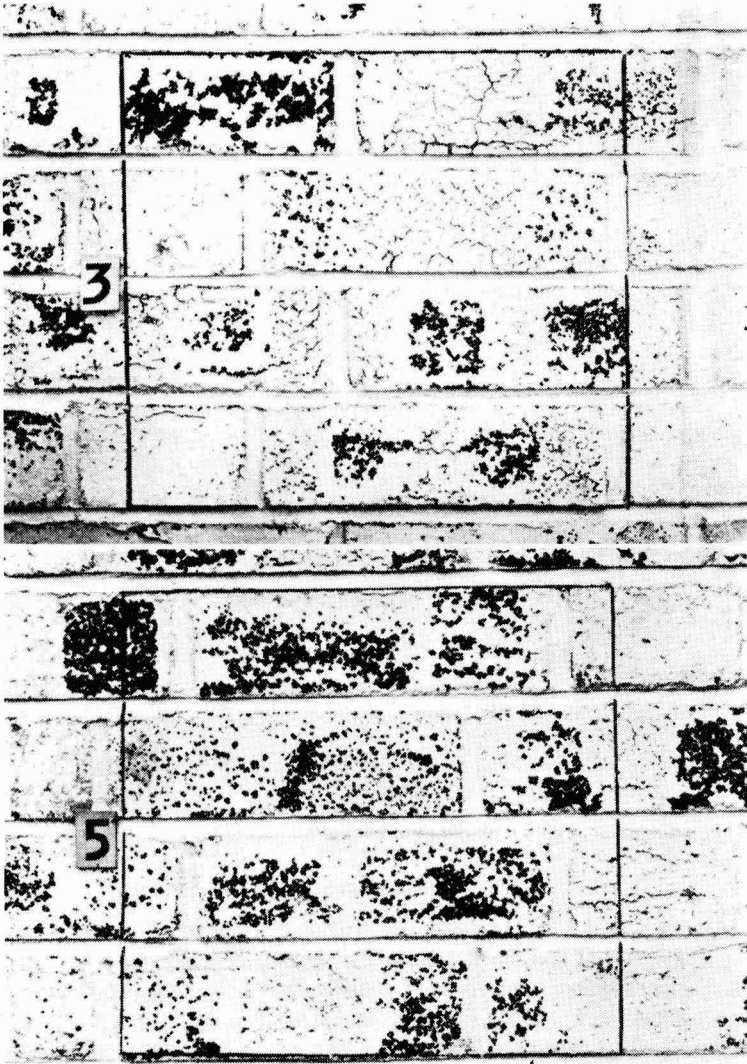
Fig. 4. Test wall at 3 years, showing failure on bricks:
