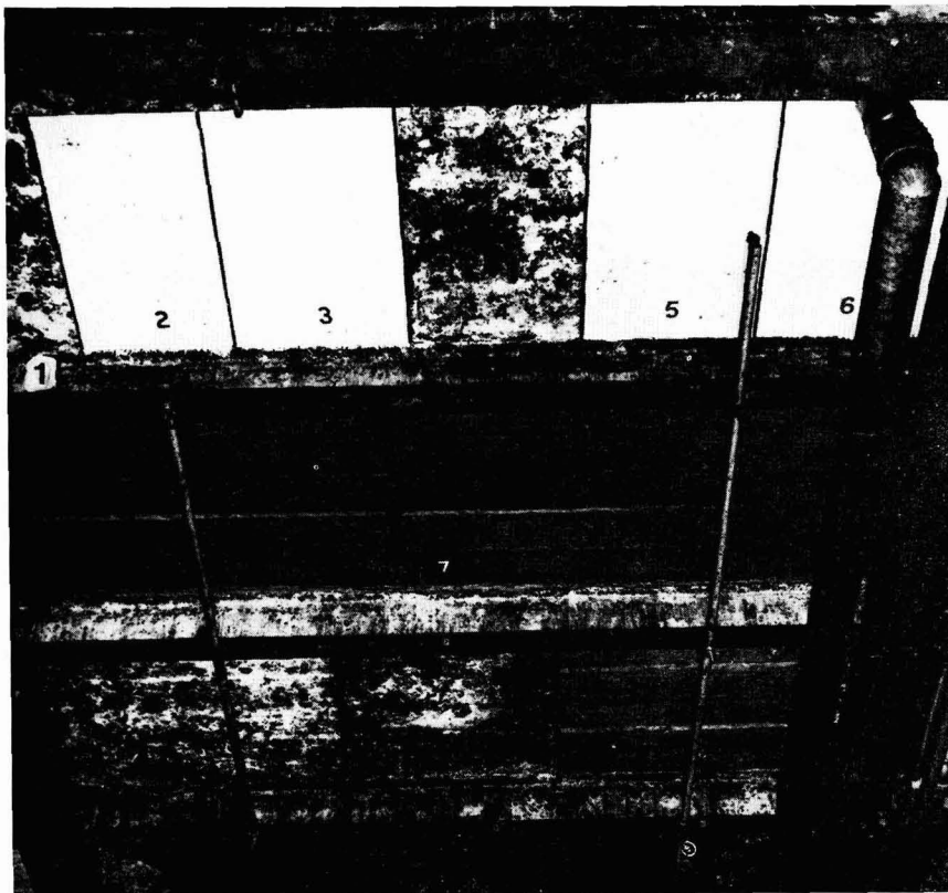
Fig. 3. Test area on ceiling over bottle washing machine in brewery, 13 months after painting
