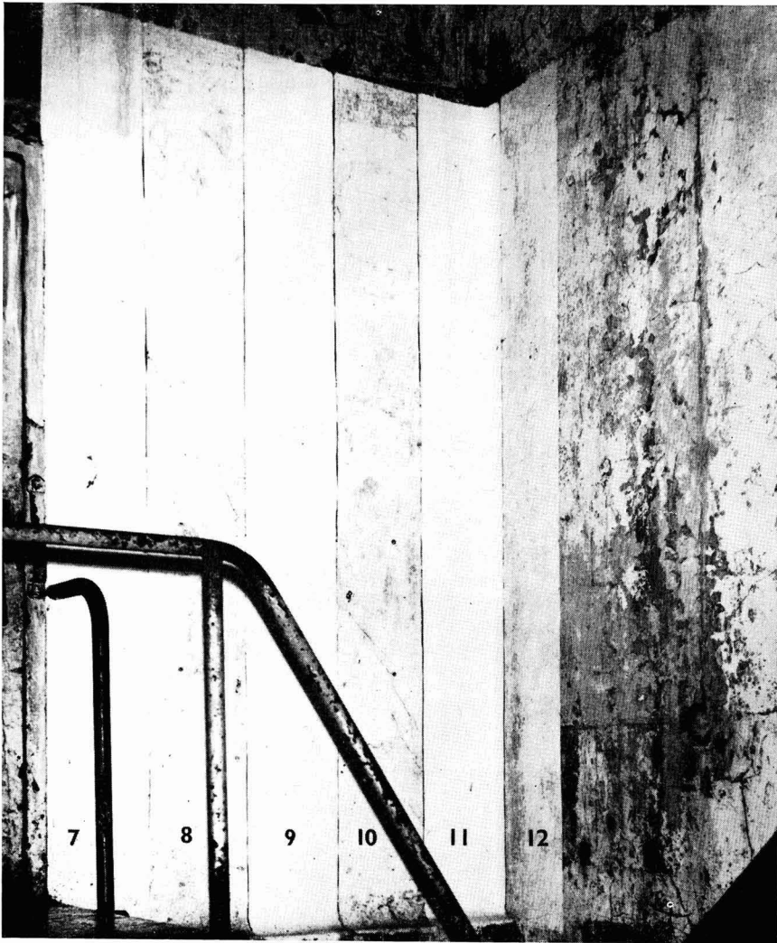
Fig. 5. Test area on wall in cold room of brewery, 5 months after painting Formulations 7, 9, 11 contain TMTD; others are blanks
