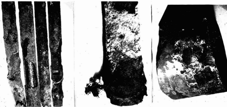
Fig. 2. Examples of corroded pipes and damaged wrappings and coatings
