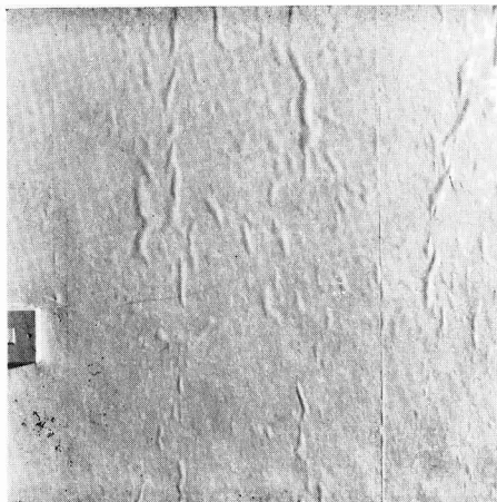
Fig. 2. Blistering on a treated wallcovering using paper as the substrate
