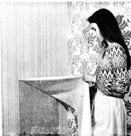
Fig. 3. A synthetic wallcovering system which is still dry strippable after being hung for a number of years
