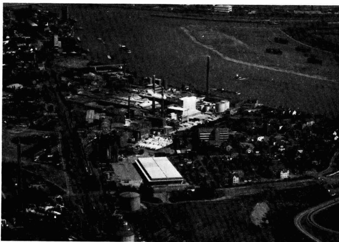
An aerial view of the Sachtleben Chemie GmbH plant at Duisburg-Homberg am Rhein
