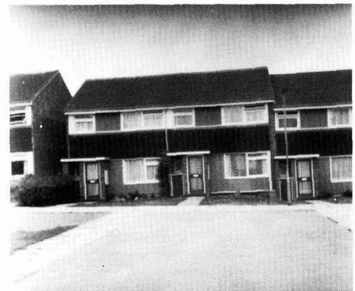
Coated plywood as a cladding, complimenting tiles and providing ground level impact resistance.
