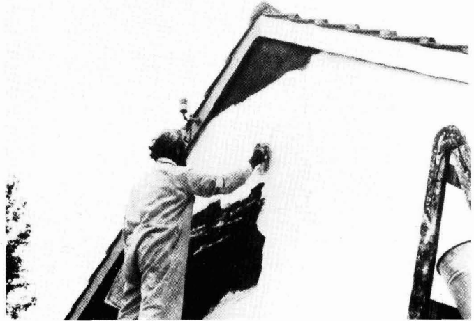
Permoglaze Thermarend being applied to a wall by a normal plastering technique
