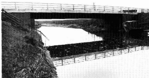
Figure 3. The Iden Bridge
