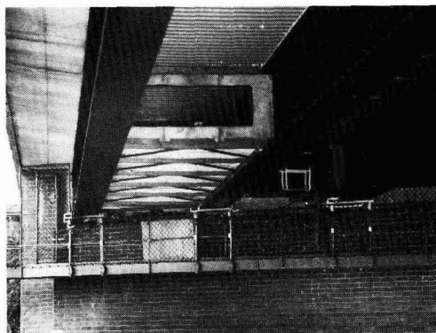
Figure 4. The Iden Bridge showing wooden boxed enclosure with plastic window
