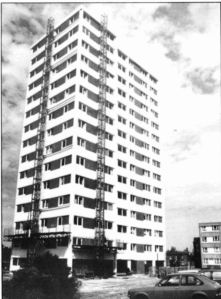
Flats in Sefton refurbished by Accrete using Bayer's Desmodur/Desmophen (DD) polyurethane resins as a basis for the coating.
