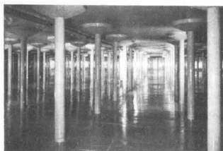
Epoxy coatings used to protect an underground water reservoir.
