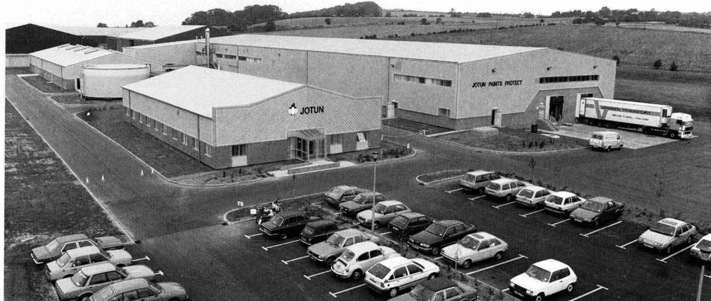
The new Jotun-Henry Clark marine and industrial coatings plant at Flixborough.
