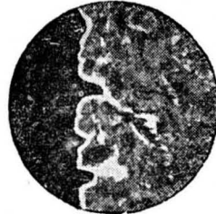
The same surface after the first coat of AQUELLA has been scrubbed into it, showing how the deep fissures have become filled and stopped.
