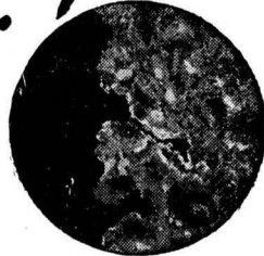
Sectional view of a masonry surface showing the porous condition due to weather erosion.
