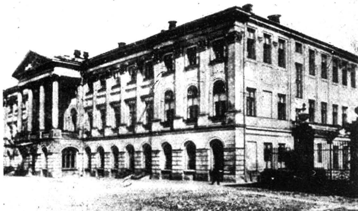
Fig. 17. The University building, Warsaw.
