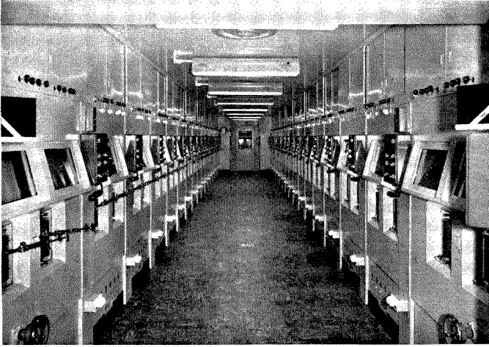
FIG. 2.—Operating aisle of remote laboratory.
